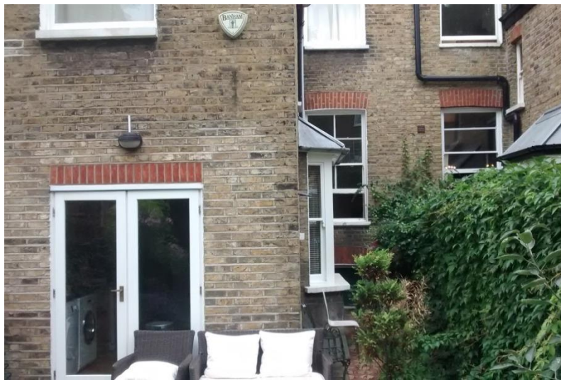
Image 2: Photograph of the Rear of the Application Site
